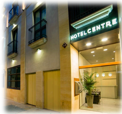
Hotel Centre Reus *** http://hotelcentrereus.com/home/
